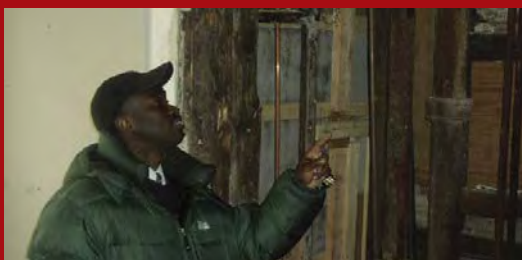
Kitchen under construction.
