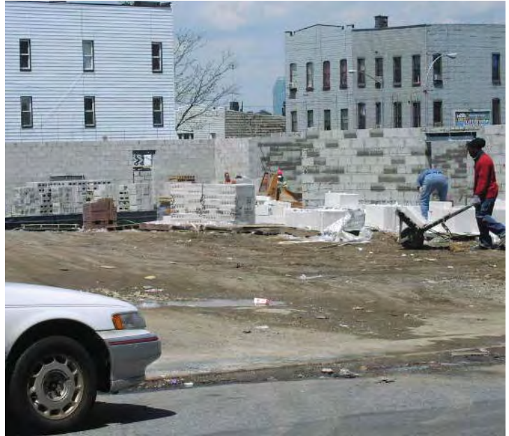
Early stages of construction
