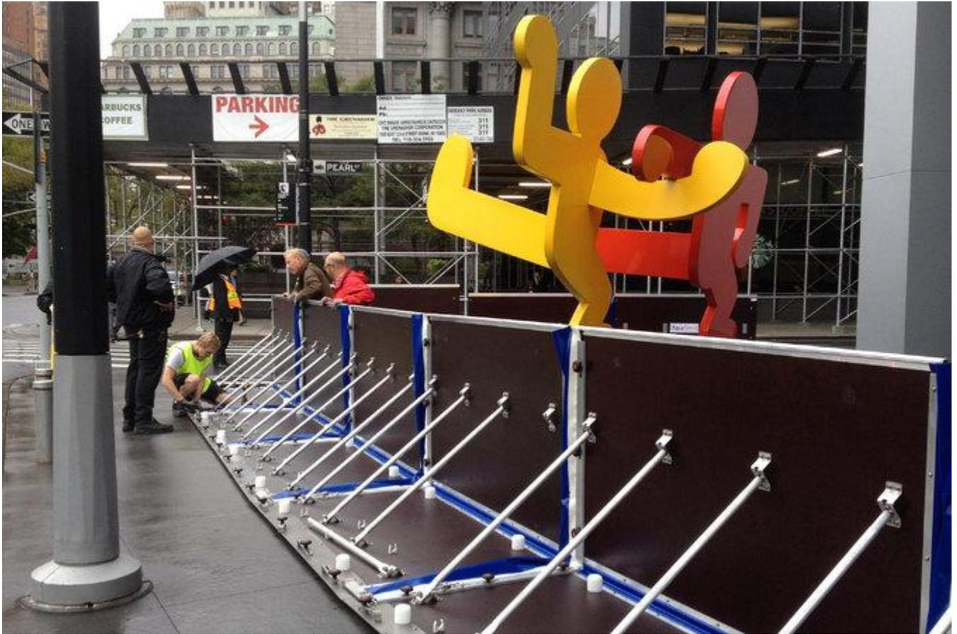
An example of an AquaFence, a deployable flood barrier. Panels can be from four to seven feet tall. Credit AquaFence
